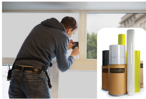
PDLC Retrofit Film Installation; PDLC Film Rolls
