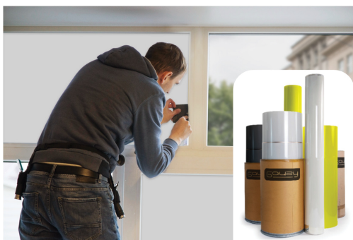
PDLC Retrofit Film Installation; PDLC Film Rolls
