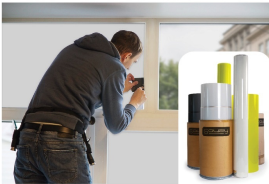
PDLC Retrofit Film Installation; PDLC Film Rolls
