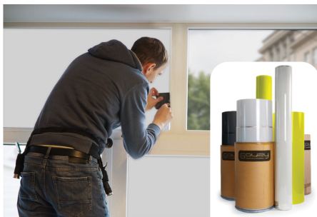
PDLC Retrofit Film Installation; PDLC Film Rolls
