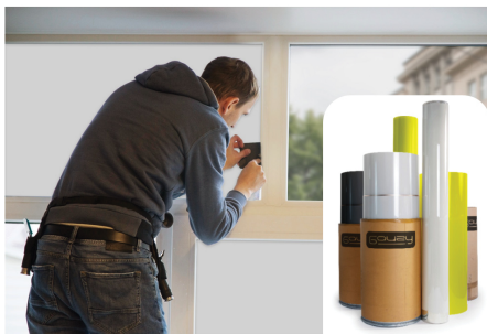
PDLC Retrofit Film Installation; PDLC Film Rolls
