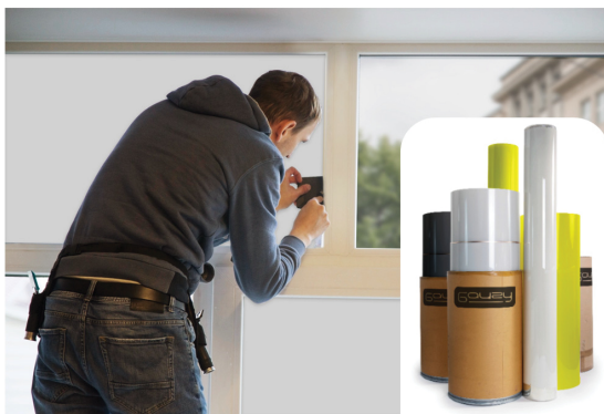
PDLC Retrofit Film Installation; PDLC Film Rolls
